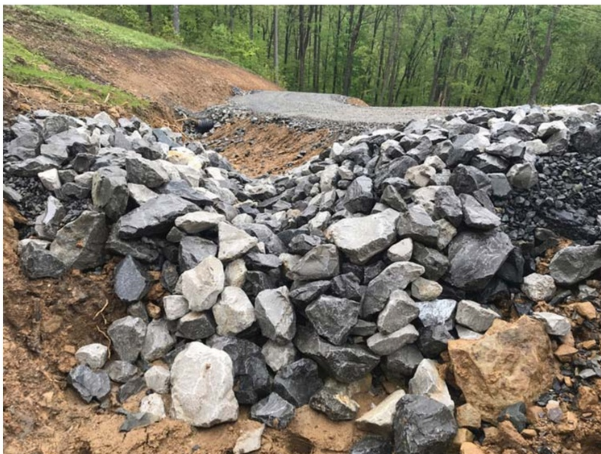
A rock check disperses water that would run downhill and erode the mountainside if not interrupted. The image was stored as a Best Management Practice in the software system.
